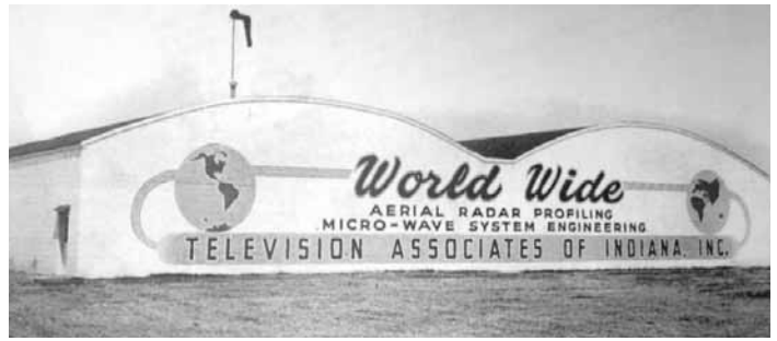
The Eddy hanger at Phillips Airport.
